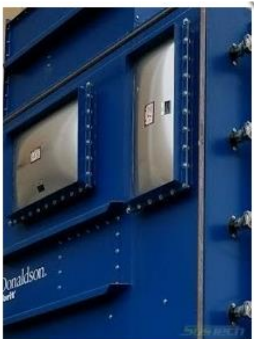
Explosion panels on dust collector.
